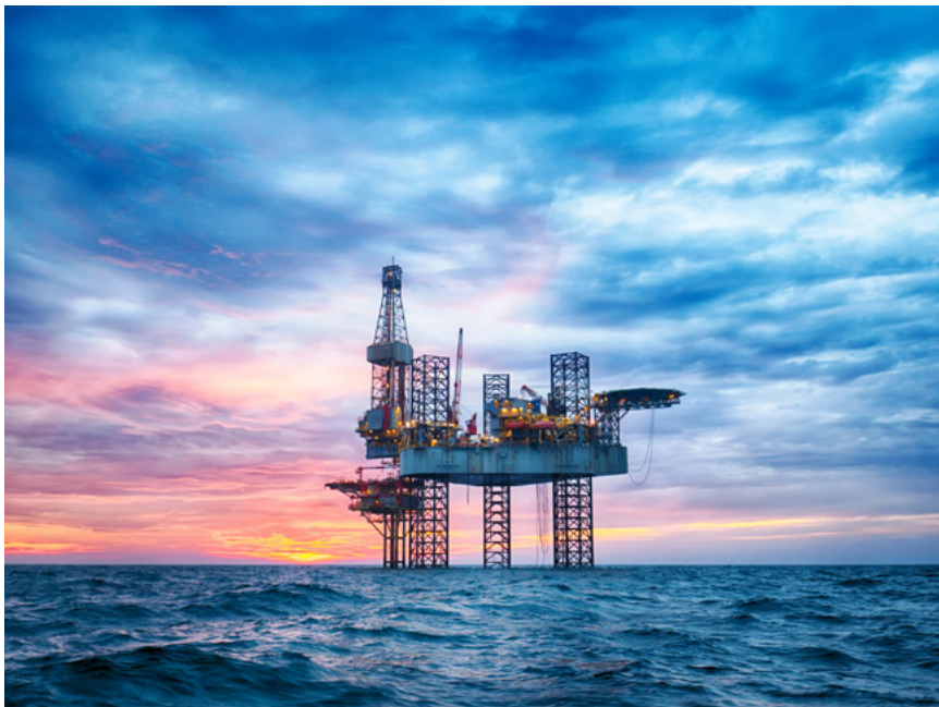
Offshore gas platform
